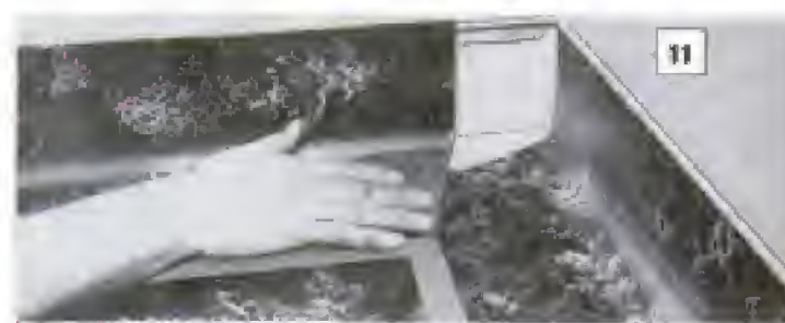
Figs. 11 and 12 show how an inside corner is cut and fitted when metal or plastic corners are not used
